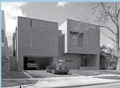
E-16 Southgate House
